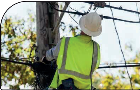
Installation of Arial OpC fibre Cable.
