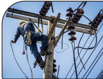
Installation of Overhead lines.
